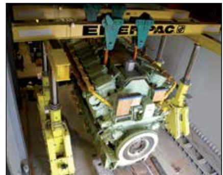
Generator Installation at the Owen Springs Power Station
