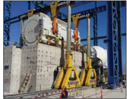
Turbine and Generator Installation at a new Power Plant in Libya
