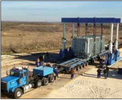
Transformer Installation with a Hydraulic Gantry
